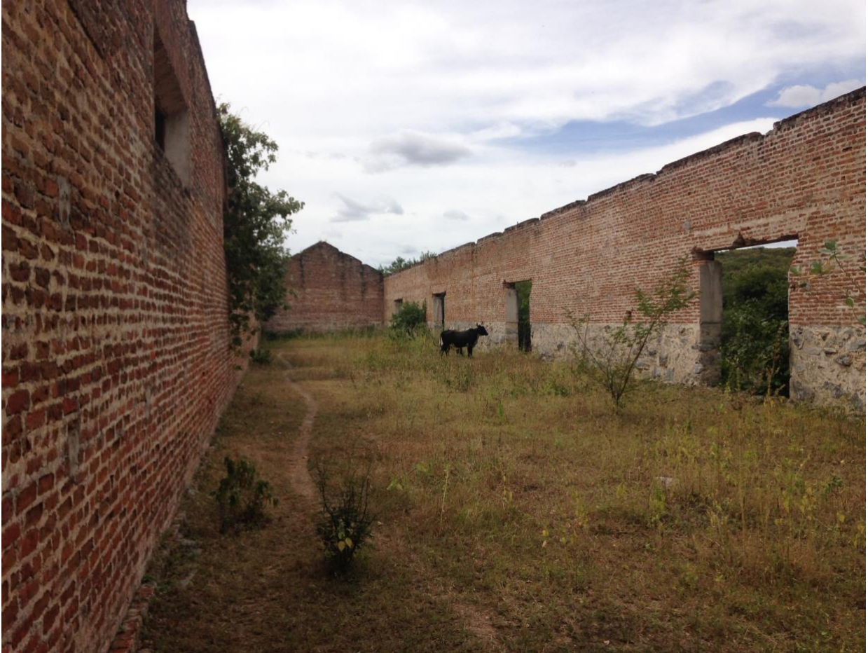
Image 1: Remaining walls from the hospital facilities at Campo do Patú, Senador Pompeu, CE. Photo by Laura Belik
